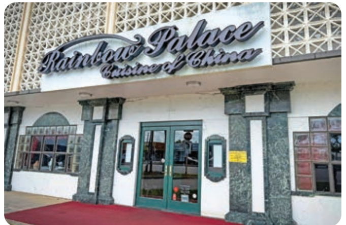
PHOTO PROVIDED BY CITY OF FORT LAUDERDALE
