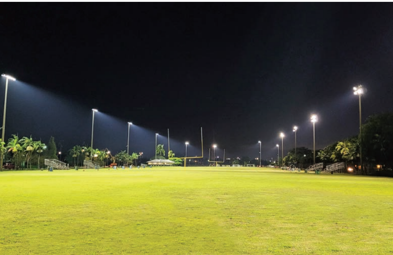
Lights on the left have been upgraded, resulting in reduced glare and more direct lighting with less spillage into the surrounding area.
