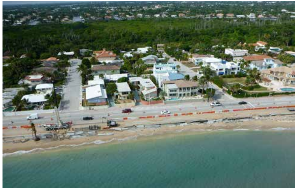
Fort Lauderdale Beach erosion in November 2012.
